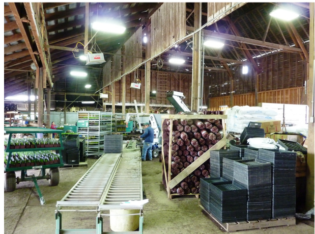
Blooming retrofitted lighting in their barn, offices, shop and lunch room.
